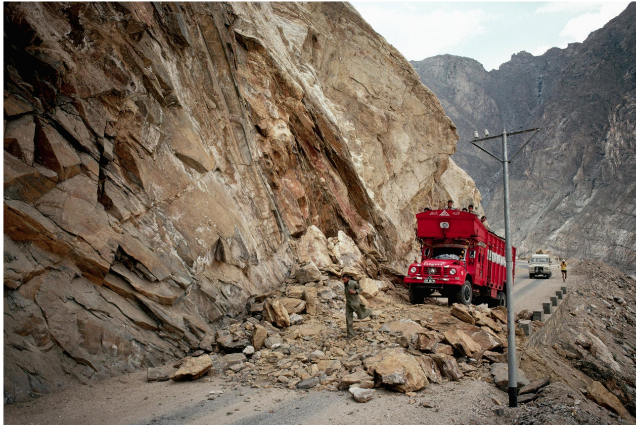
Rockfall Karakorum Highway – unsecured rockcuttings
