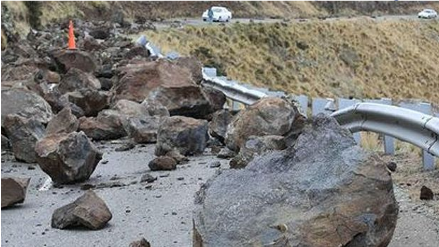
Rockfall after earthquake in NZ summit road, Port Hills February 2011
